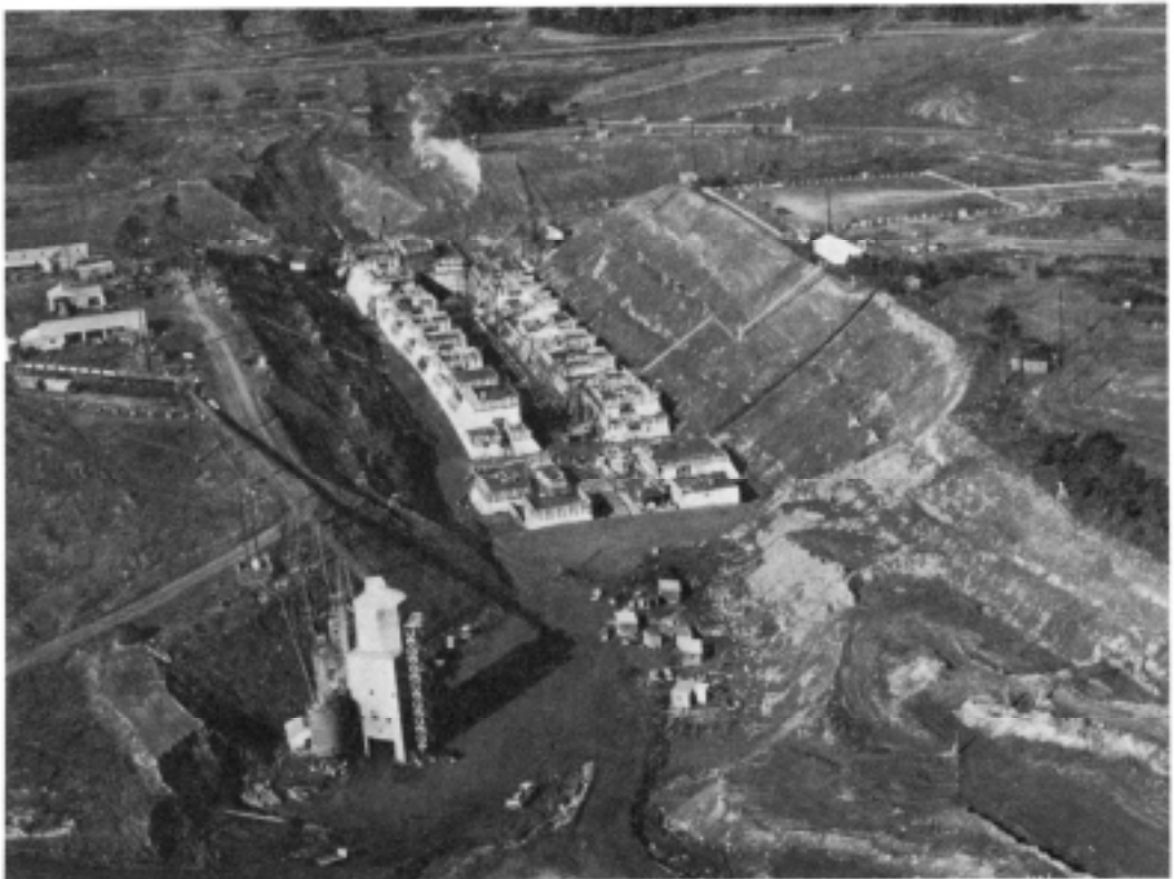
Lock and related construction activity, September 1956.
