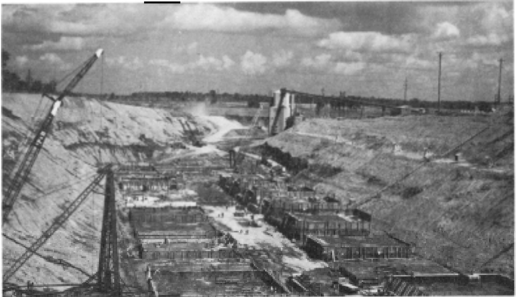
Construction, looking eastward, August 1956.
