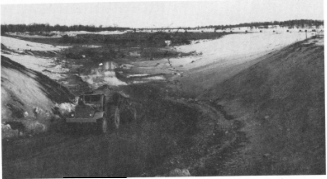
Excavation, from the west end, February 1956. A bottom-dump Euclid in the foreground.
