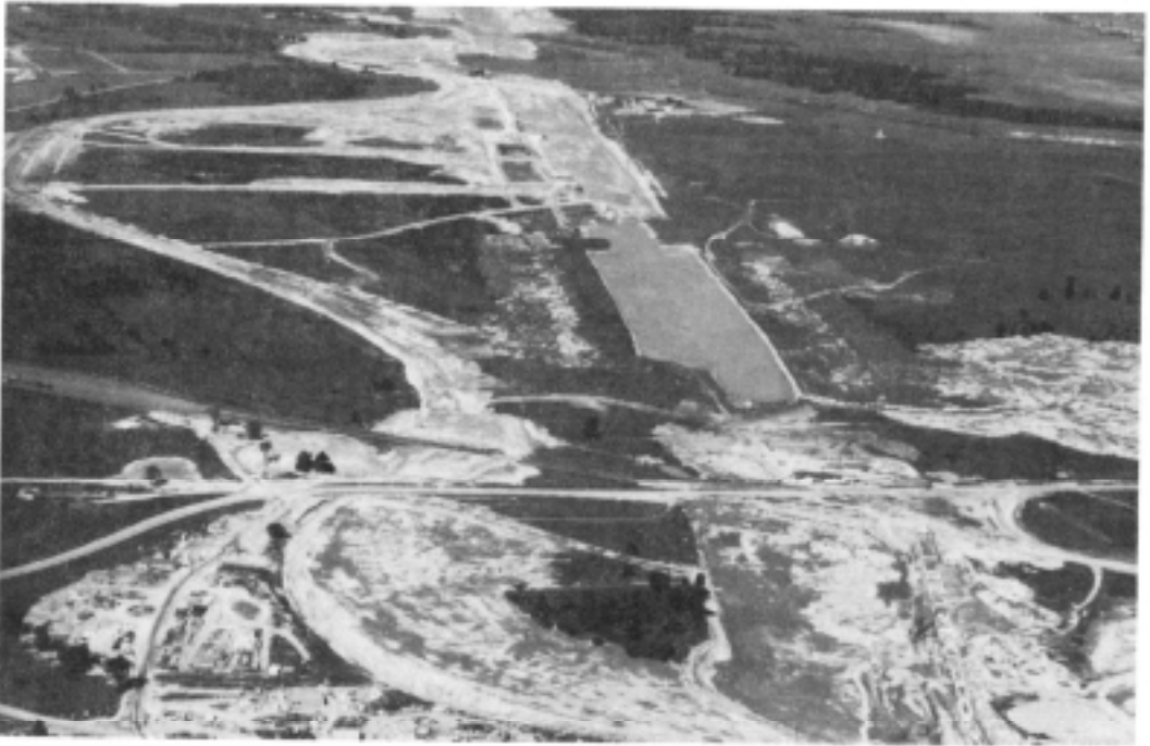
The project, July 1957.
