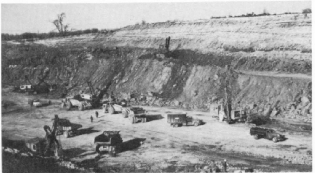
Shovels excavating, January 1956.
