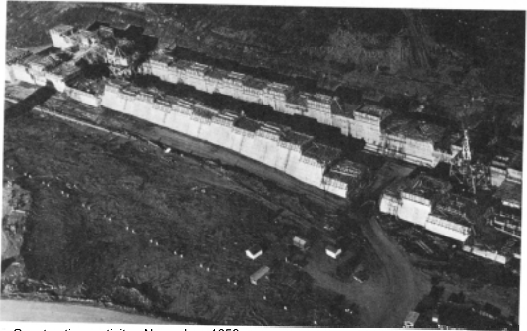
Construction activity, November 1956.
