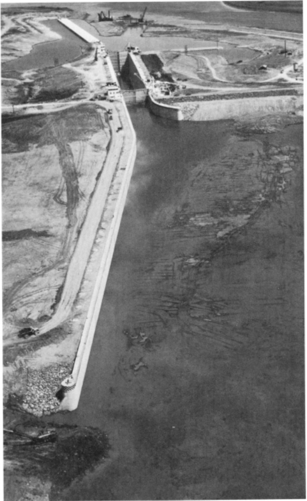
Removing the plugs, May 1958.
